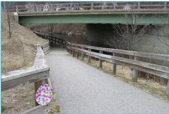
15. RAIL TRAIL UNDERNEATH RT.101 AT PETERBOROUGH PLAZA
