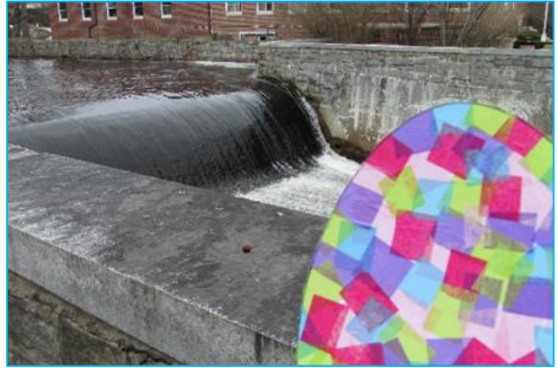
14. NUBANUSIT SPILLWAY @ PUTNAM PARK (POST OFFICE IN BACKGROUND)
